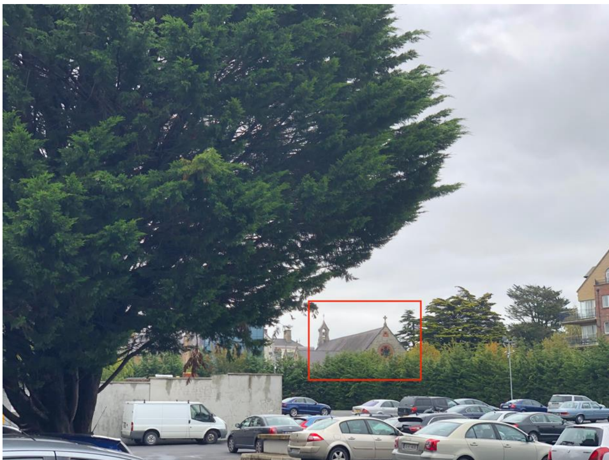
Fig. 2: View of the northern end of the car park to the rear of the Bonnington Hotel. © JFM Research
